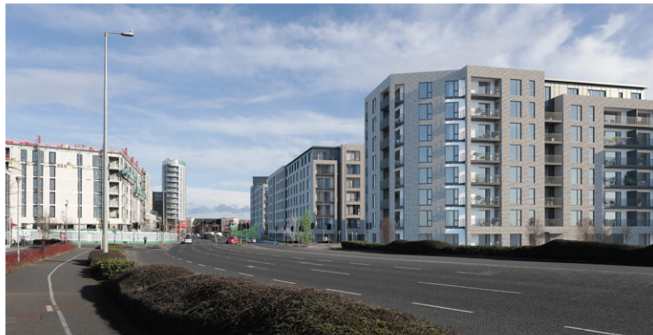
Image 24 – View along Charlestown Place Road looking East
