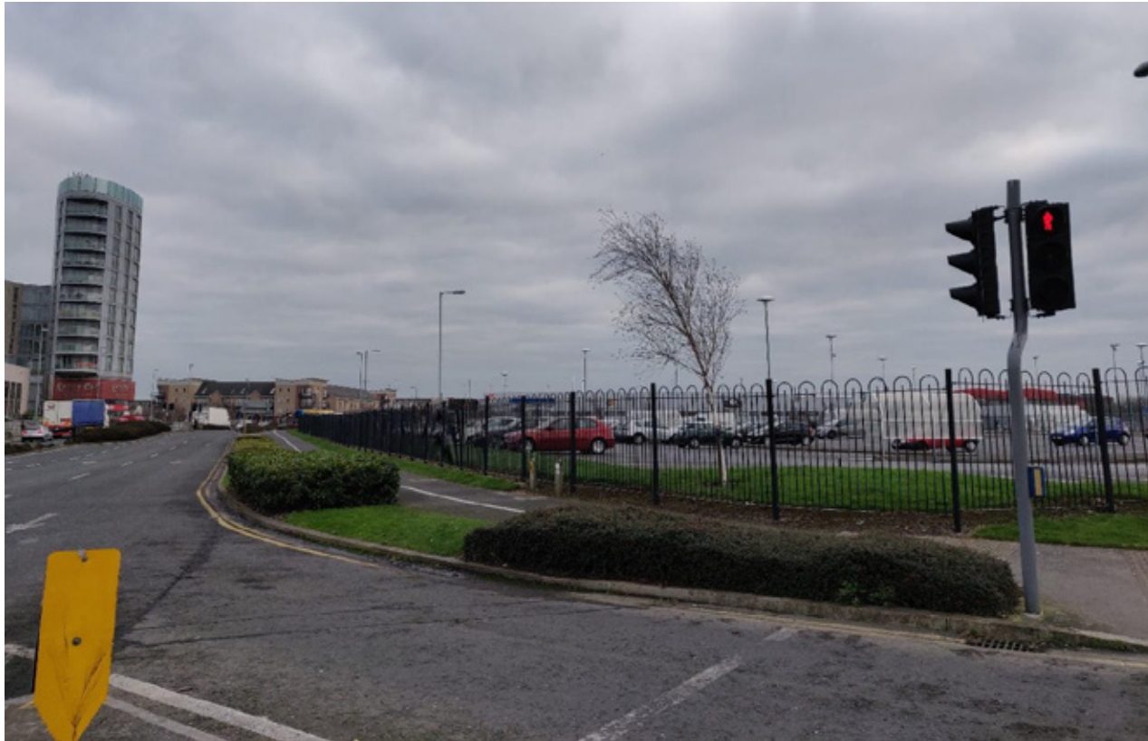
Image 2 – Site Photo looking east across site and Charlestown Place Road
